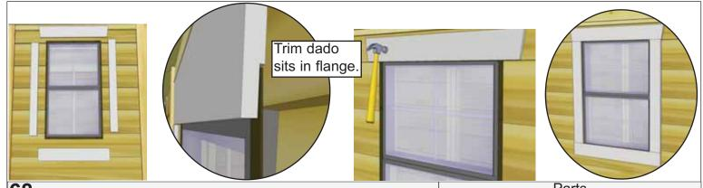
**68.** Position **4X - Window Trim** around window doing a dry run first and attach with **4 - 1 1/2" Finishing Nails** per piece. Window trim has a small dado on reverse face. Outside flange of window will roughly sit in the dado to give a better fit. Complete both windows the same.
